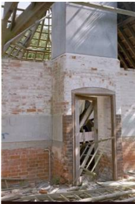
Figure 2 Barn 1 interior facing NE showing door to porch, water tank above, concrete splash-back and water pipe
