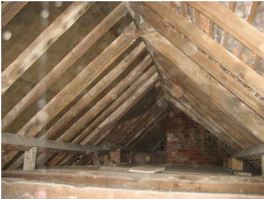
Figure 6 Roof space looking east
