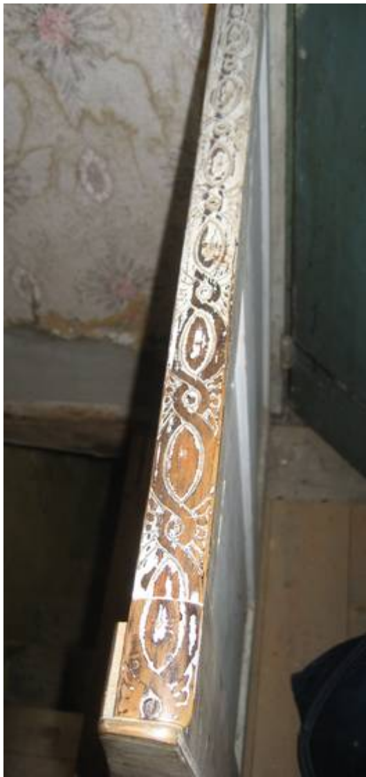
Figure 11 Carved rail at the top of the central stairway -the stairs are to the left, the landing to the right.
