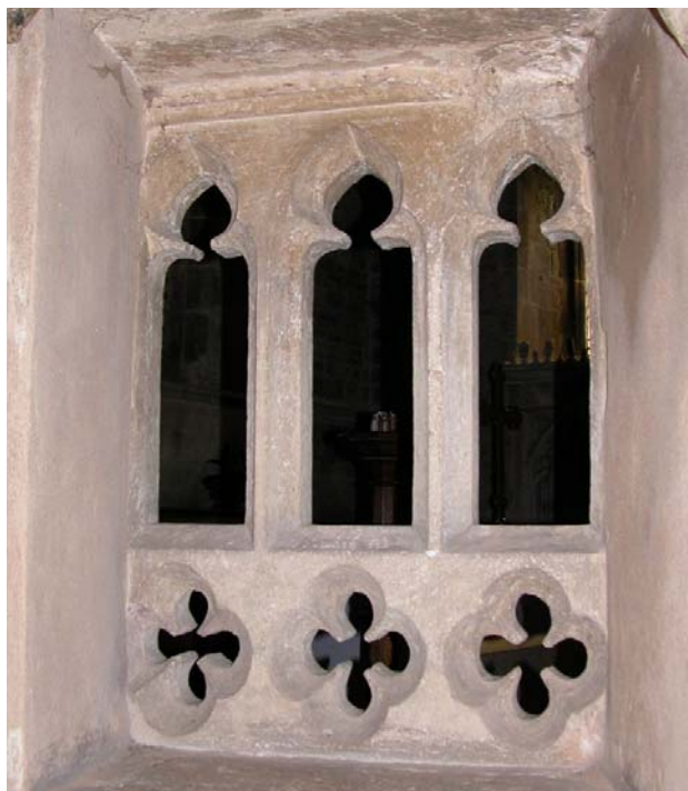
Squint window between chancel and chantry chapel in the church, Chipping Norton. The ‘candle flame’ shape is reminiscent of some recently spotted in barns around Burford
