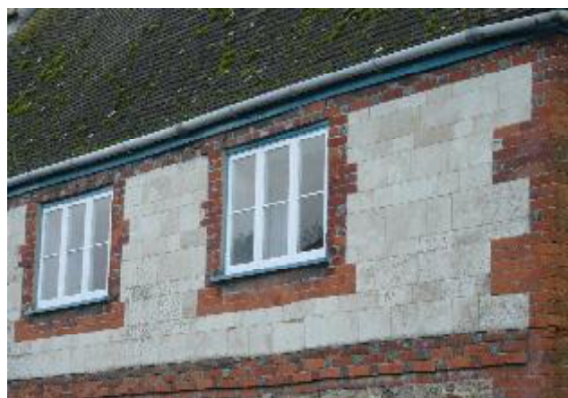
18 th C farm house with brick banding, openings and quoins
