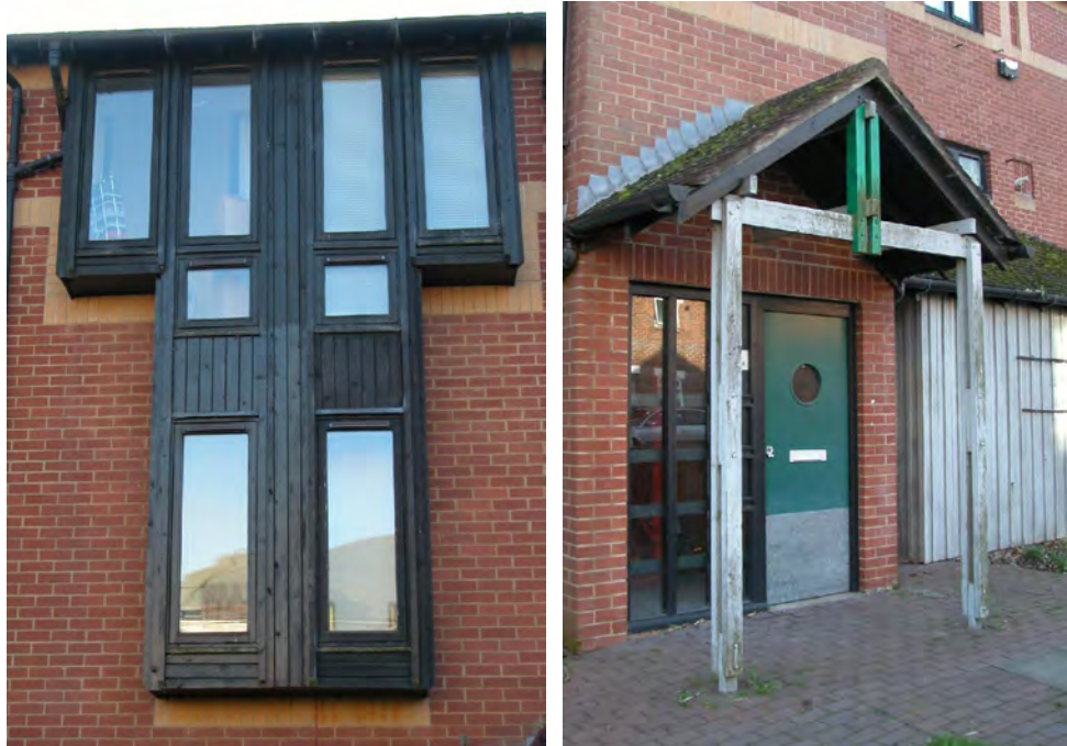
Details of windows and doorway at Abbey Place (2005)
